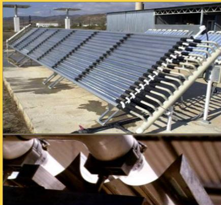
Compound Parabolic Collector
