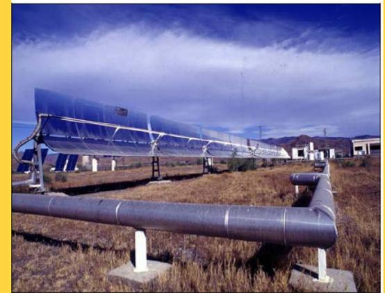
Parabolic Trough (PSA)
